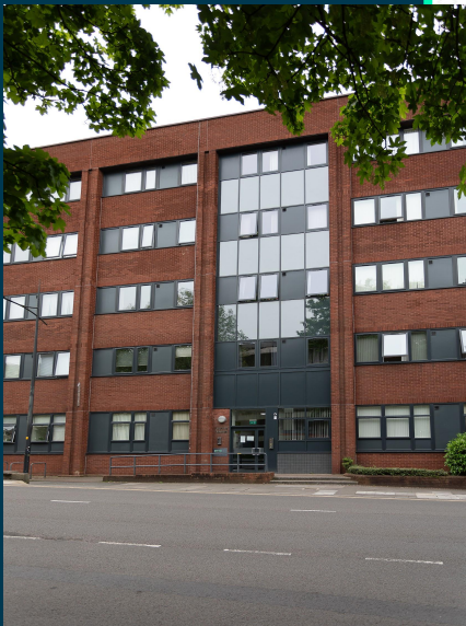
Electra House, Farnsby Street Swindon, SN1
